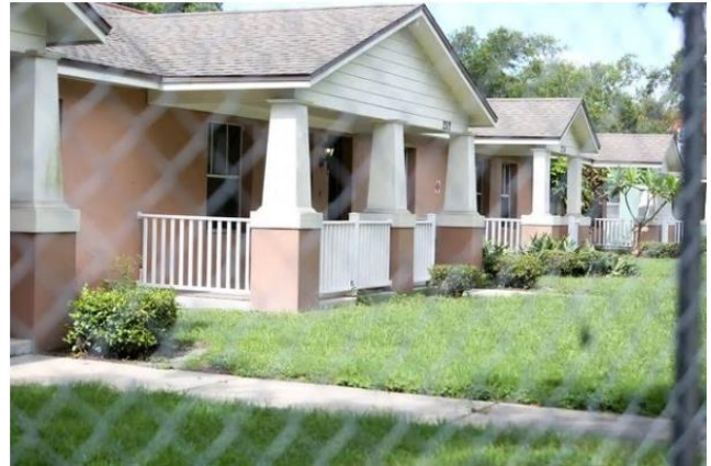
The bungalows of Jordan Park sit empty behind a gate put up to enclose the properties due to be demolished as part of the redevelopment of Jordan Park. The project is being financed through a partnership between the St. Petersburg Housing Authority and Norstar Development.
